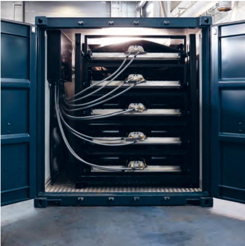
The energy storage is based on used lithium-ion batteries from the automotive industry's electric vehicles. Reusing them in energy storage facilities almost doubles the life of the batteries. The potential in the systems is great and there are many areas of application. Initially, BatteryLoop is focusing on solutions for properties, ports and logistics centers.
