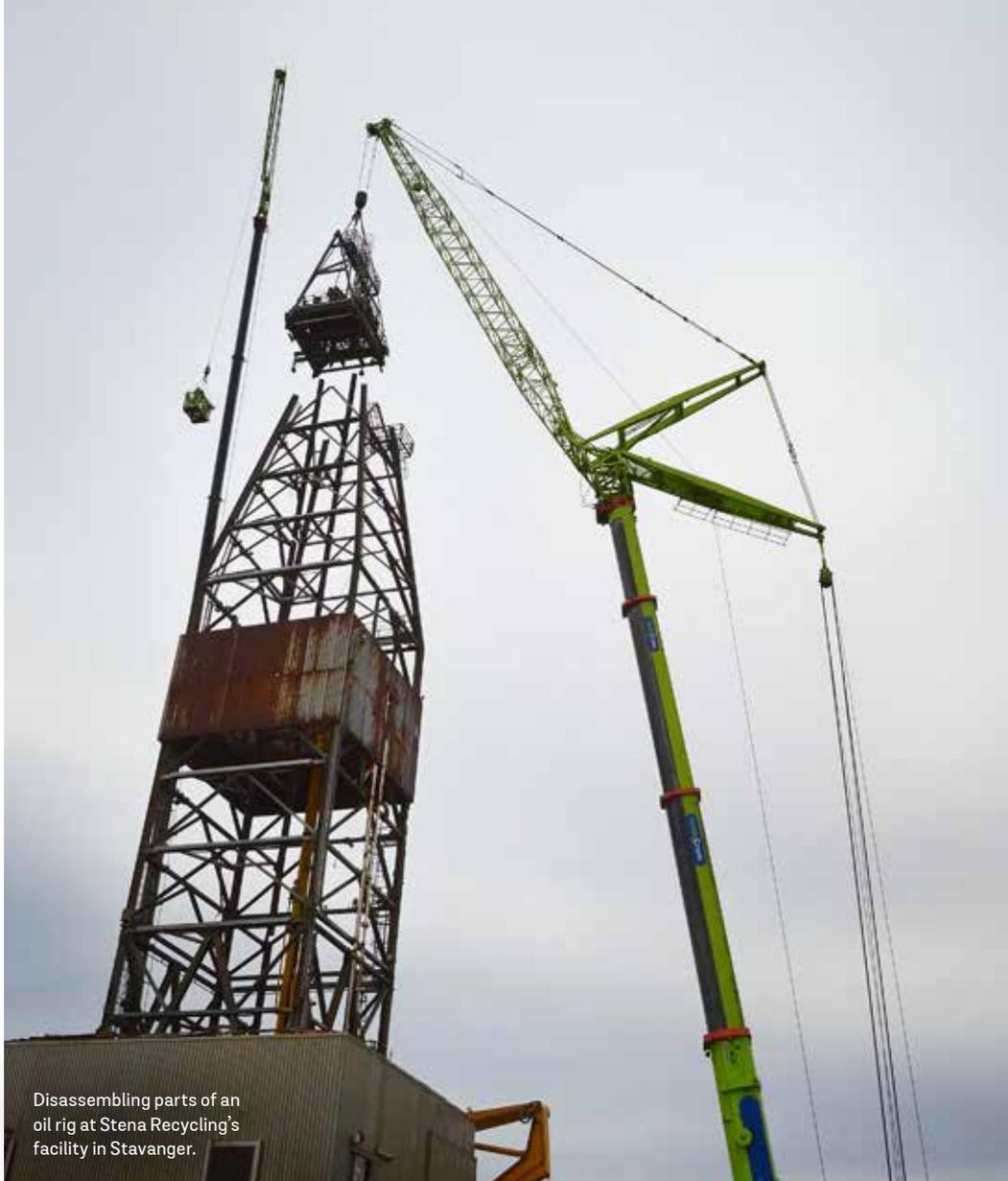
Disassembling parts of an oil rig at Stena Recycling's facility in Stavanger.
